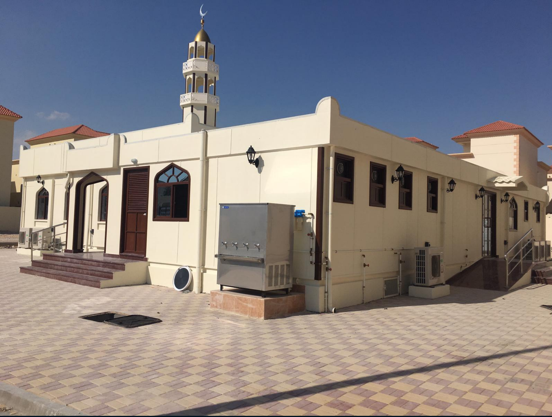
Installation of Pre-Fabricated Mosque for Ministry of AWAQF
